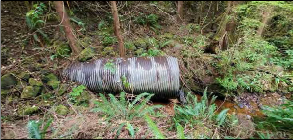
Photo 29. The Western Stream enters the southwest portion of the property from a large diameter culvert that crosses Peninsula Road. Showing culvert outlet.
