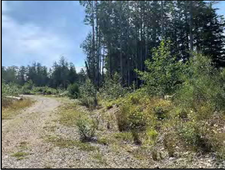
Photo 27. The road that terminates at the northern tip has ditching alongside the road that drains toward the foreshore setback.
