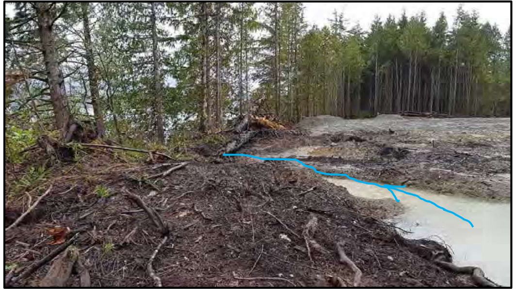
Photo 10: Cleared section of site within 30m foreshore buffer. 30m foreshore riparian buffer to be re-established.
