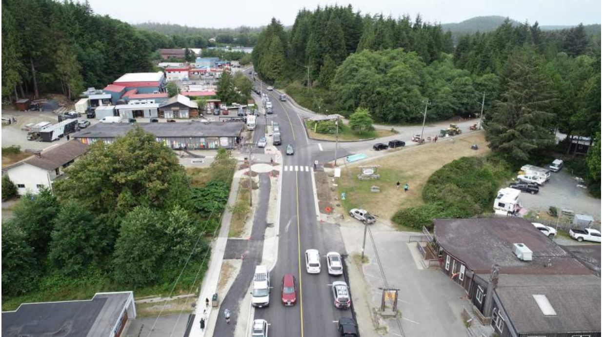
Photo #5 – Shouldering & Growing Medium Installation Ongoing
