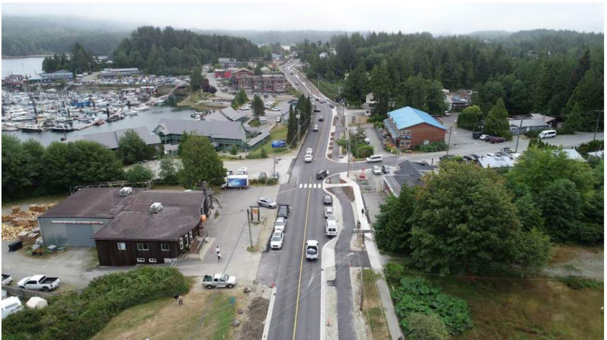
Photo #8 – Shouldering & Growing Medium Installation Ongoing
