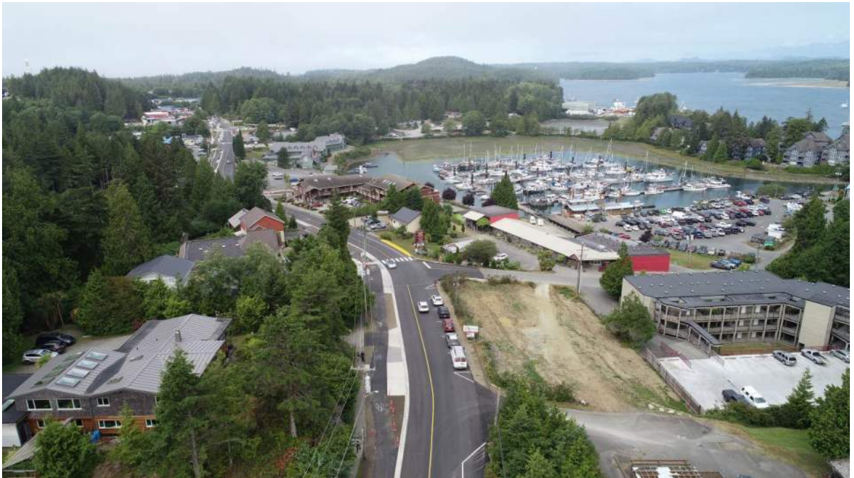
Photo #2 – Shouldering & Growing Medium Installation Ongoing
