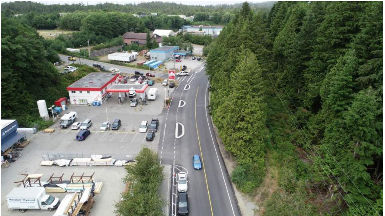
Photo #6 – Shouldering & Growing Medium Installation Ongoing
