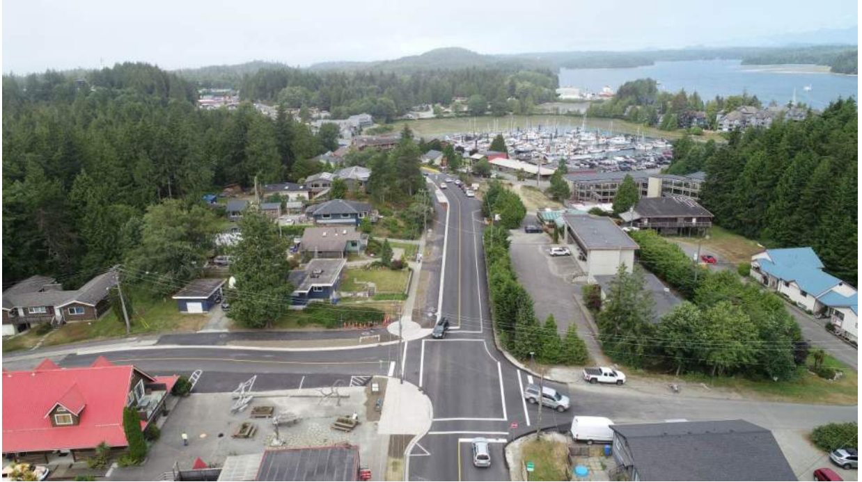
Photo #1 – Shouldering & Growing Medium Installation Ongoing
