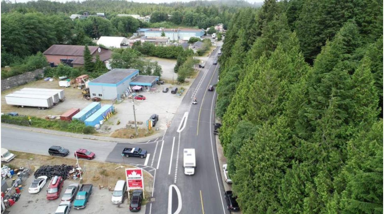
Photo #7 – Shouldering & Growing Medium Installation Ongoing
