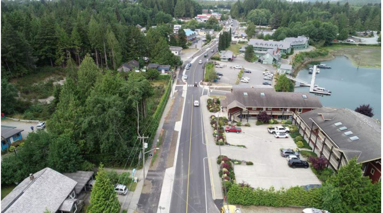
Photo #3 – Shouldering & Growing Medium Installation Ongoing
