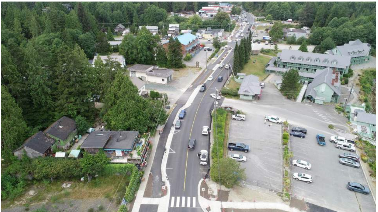
Photo #4 – Shouldering & Growing Medium Installation Ongoing
