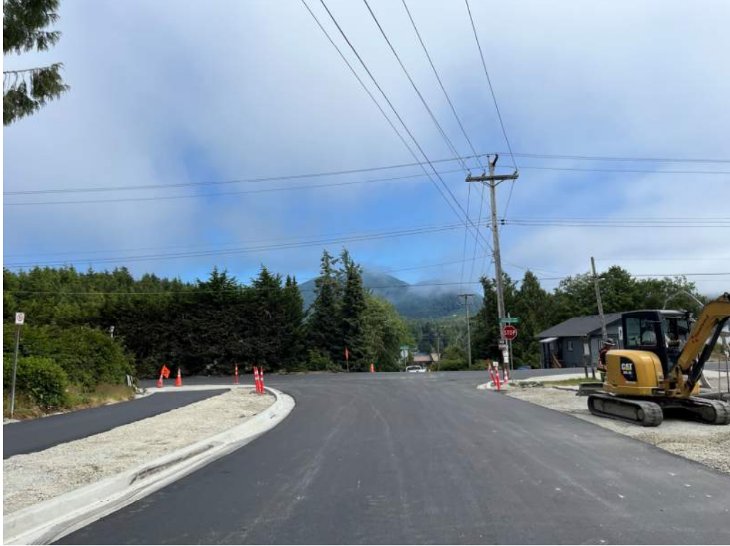
Photo #7 – Roadway Paving (Top Lift) Completed
