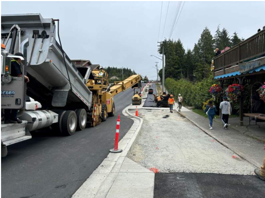
Photo #2 – Bike Tracking Paving Completed
