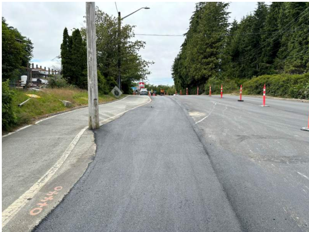
Photo #4 – Roadway Shoulder / Parking Paving Completed
