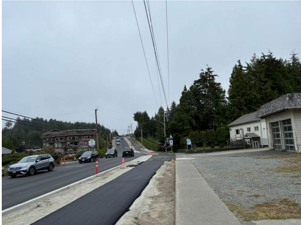
Photo #3 – Bike Tracking Paving Completed
