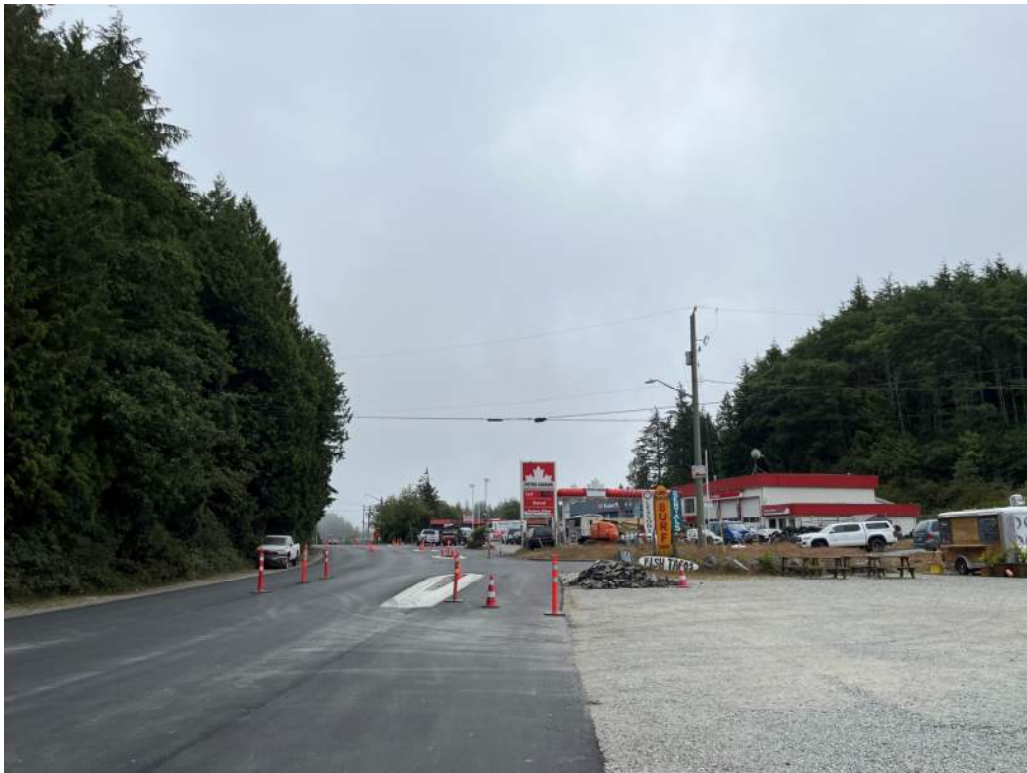
Photo #6 – Roadway Shoulder / Parking Paving Completed
