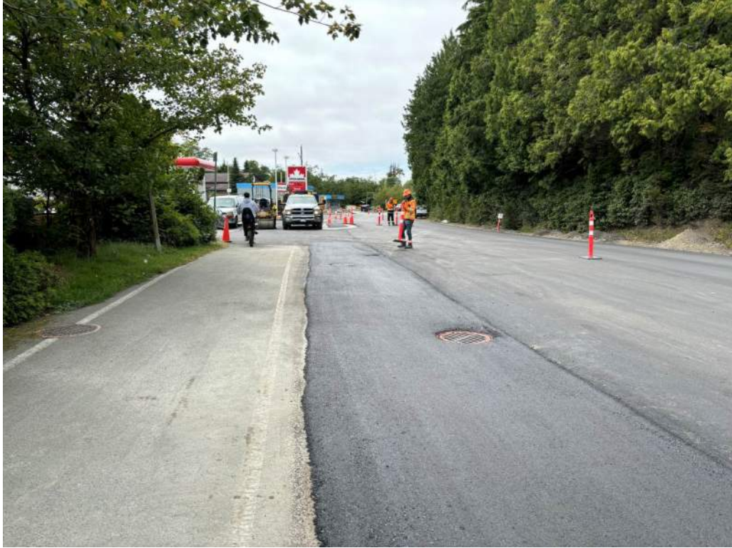
Photo #5 – Roadway Shoulder / Parking Paving Completed
