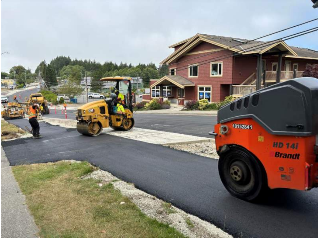
Photo #1 – Bike Tracking Paving Completed
