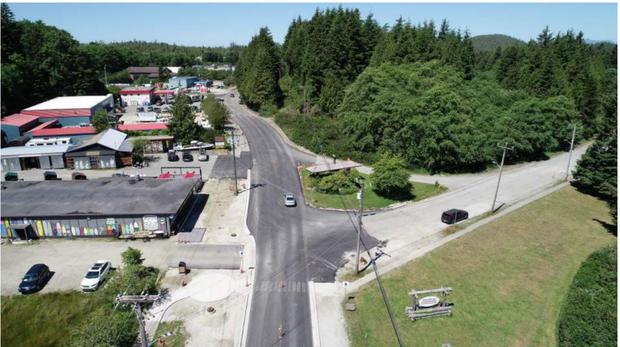
Photo #12 – Roadway Paving (Bottom Lift) Progress
