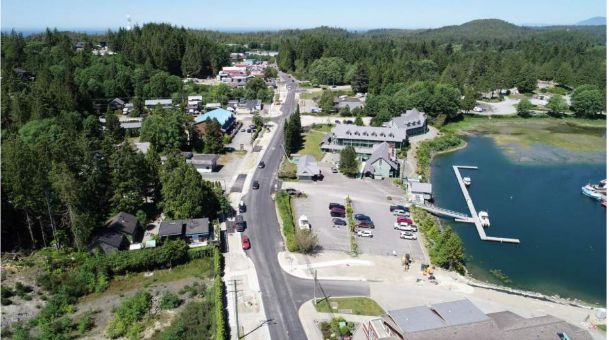
Photo #11 – Roadway Paving (Bottom Lift) Progress
