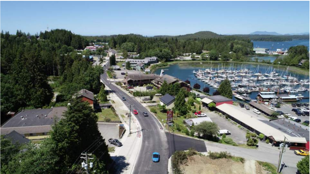
Photo #10 – Roadway Paving (Bottom Lift) Progress
