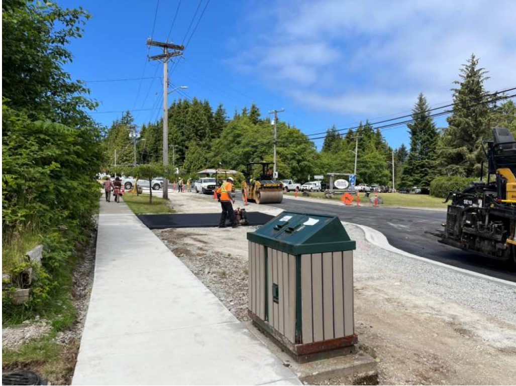
Photo #1 – Driveway Paving Ongoing
