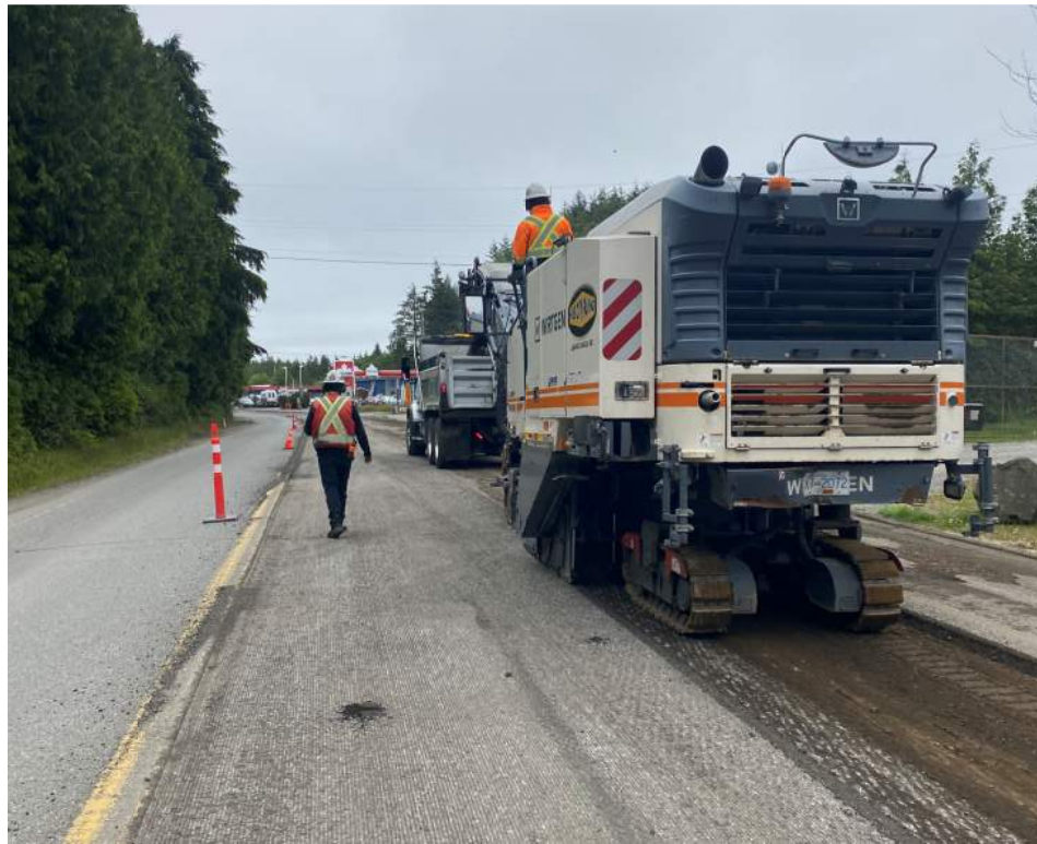
Photo #4 – Roadway Milling Completed
