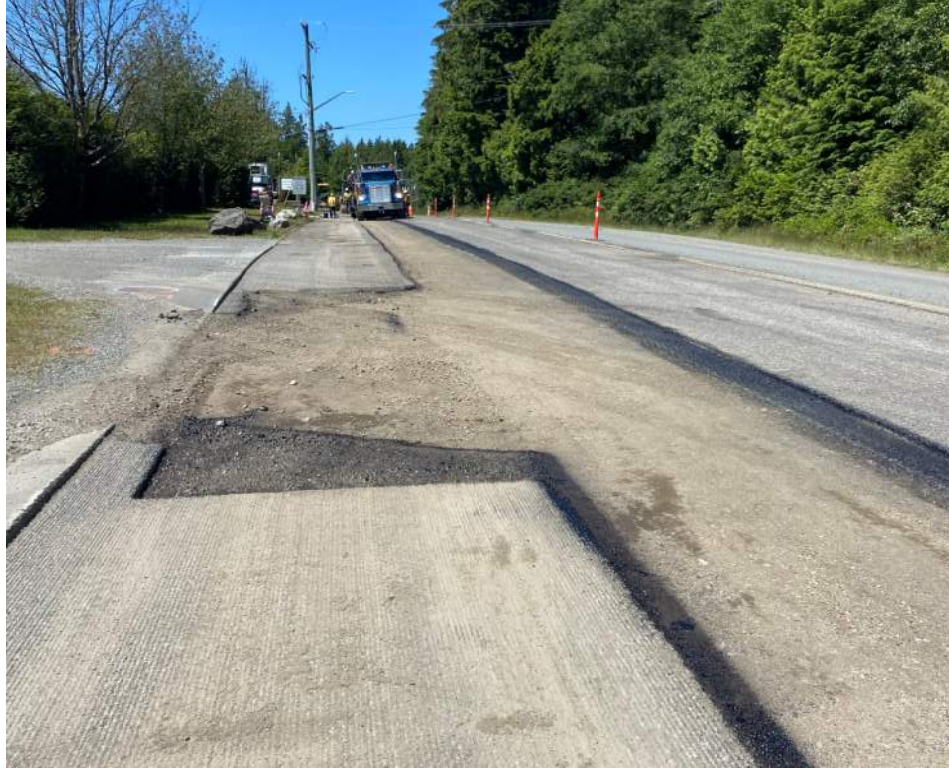
Photo #5 – Roadway Paving (Bottom Lift) Ongoing
