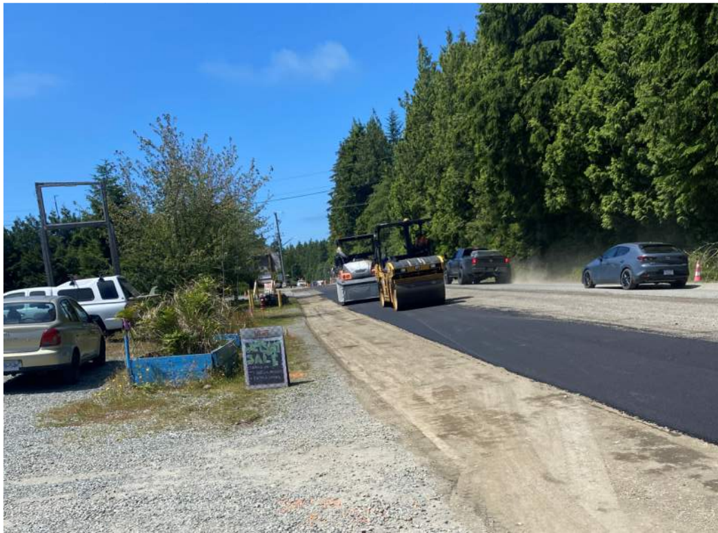
Photo #6 – Roadway Paving (Bottom Lift) Ongoing
