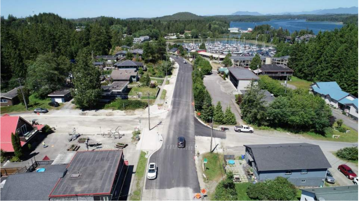
Photo #9 – Roadway Paving (Bottom Lift) Progress
