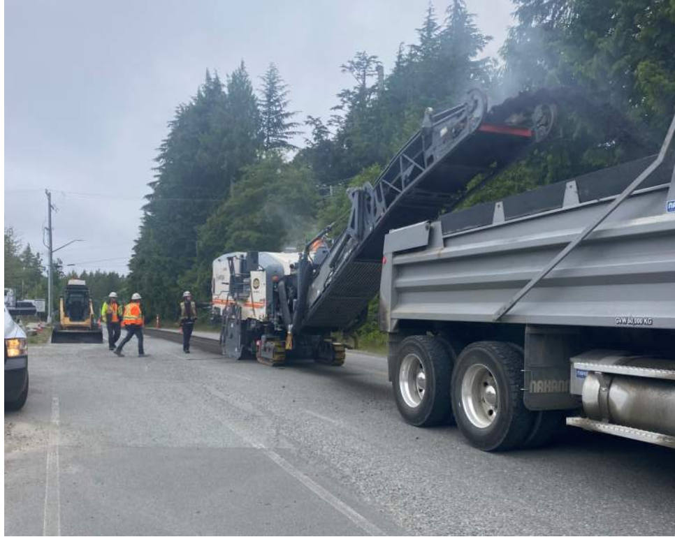
Photo #3 – Roadway Milling Completed
