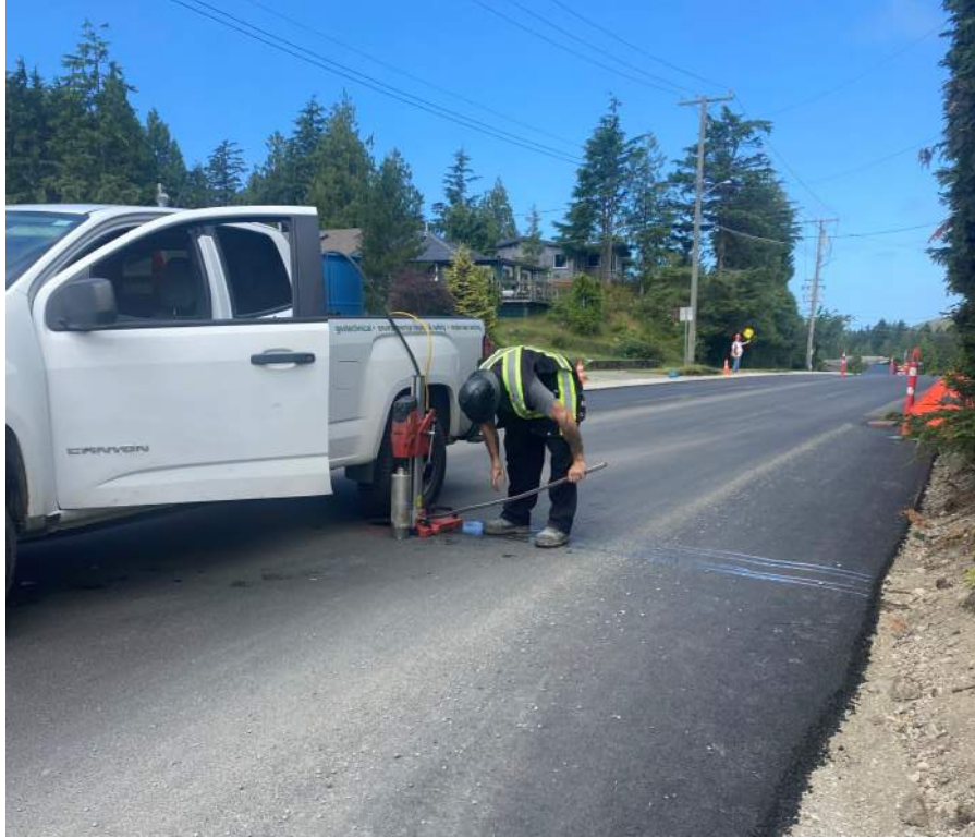
Photo #7 – Asphalt Cores for Bottom Lift Collected
