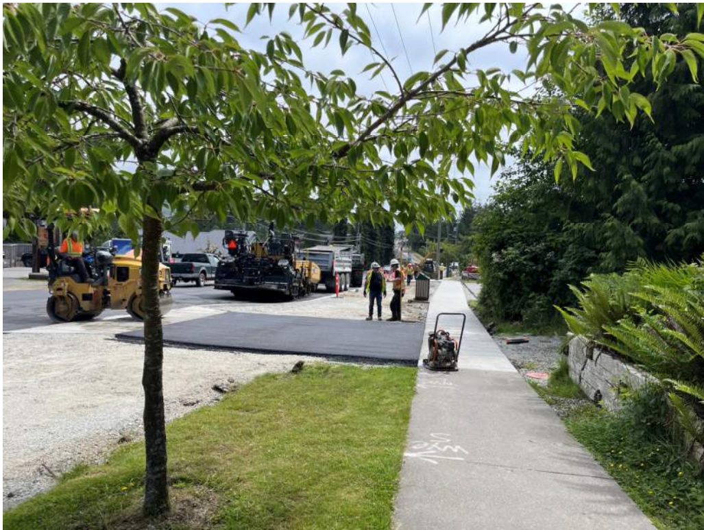
Photo #2 – Driveway Paving Ongoing
