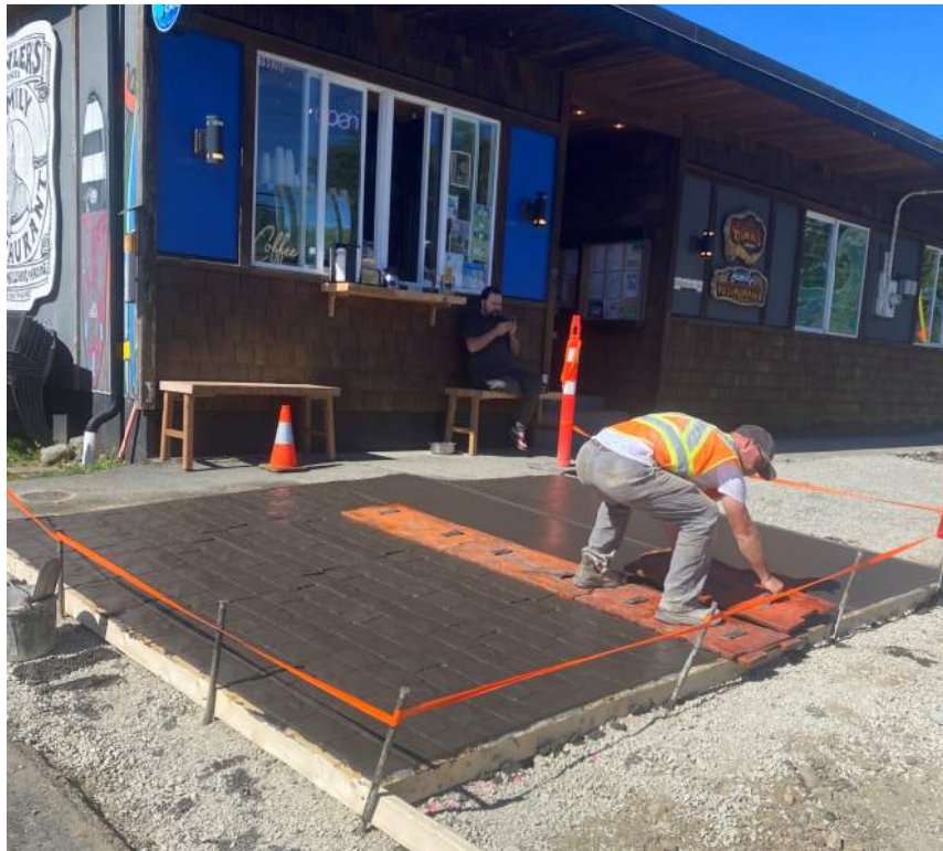
Photo #8 – Stamped Concrete In Progress
