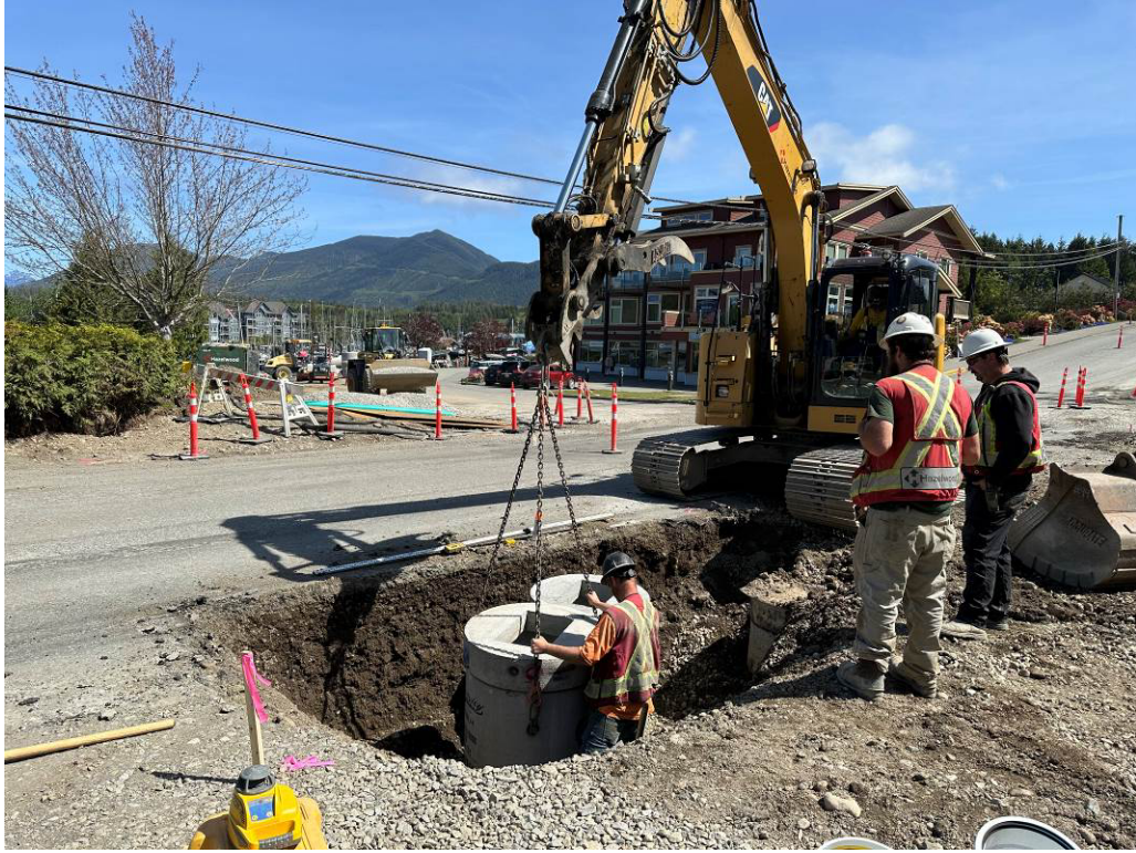
Photo #3 – Catch Basin Installations Ongoing
