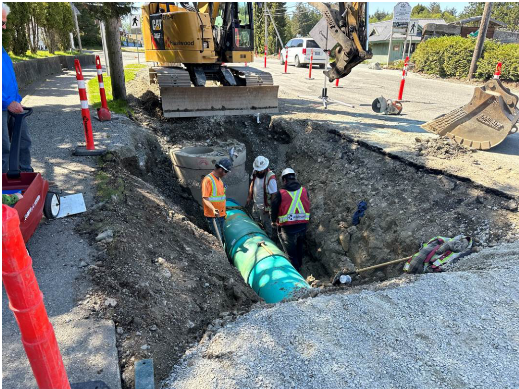
Photo #2 – Connection at DMH #5 Completed
