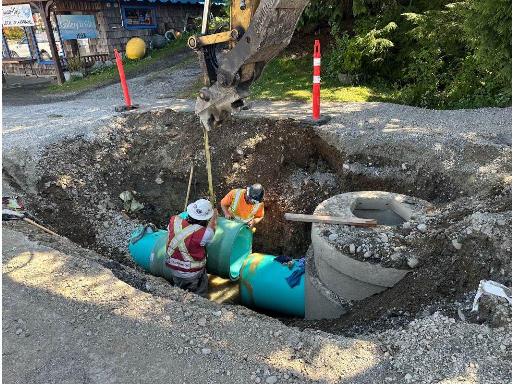
Photo #1 – Connection at DMH #5 Completed
