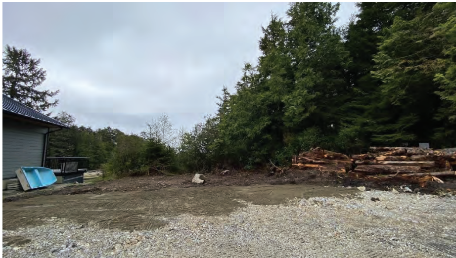
Photo 1. Looking south towards the ocean from the cleared house site that is outside of the 30 m DPA. Photo shows previously cleared area along the west side of the DPA (left) and forested portion of DPA (right).
