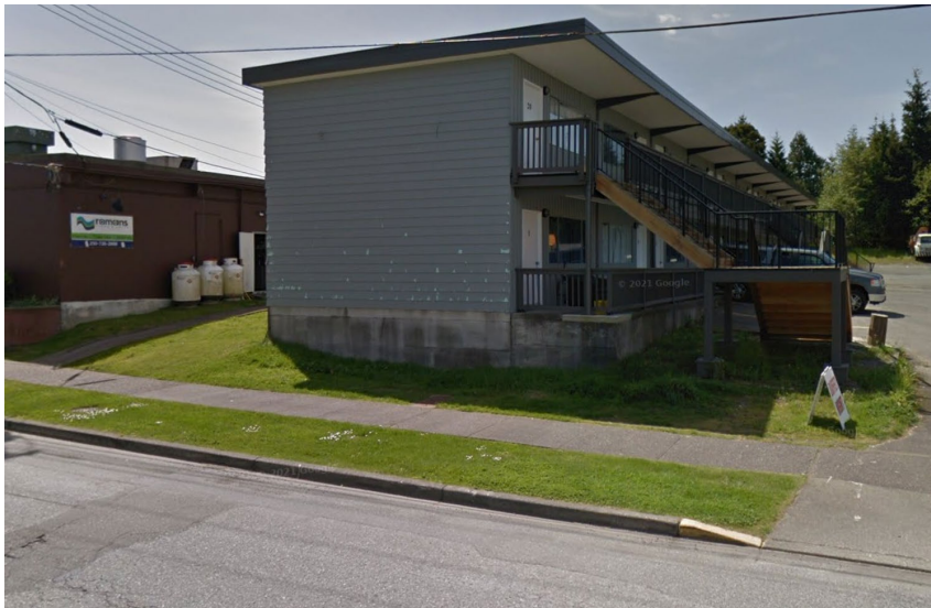
Figure 4 – Existing motel building front face
