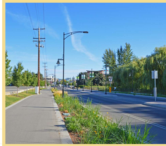
Multi-use pathway separated from the roadway with a landscaped boulevard and on-street parking (Kelowna, BC)
