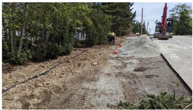
Photo #3 – Root Guard Installation Completed (Sta. 5+340 to 5+390)
