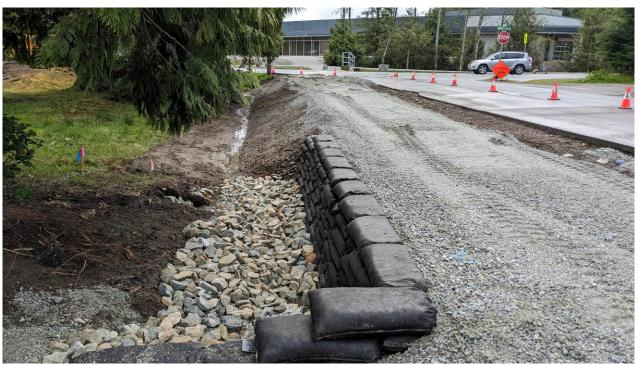
Photo #1 – Larch Road Pathway – Roadway Widening in Progress (5+500)
