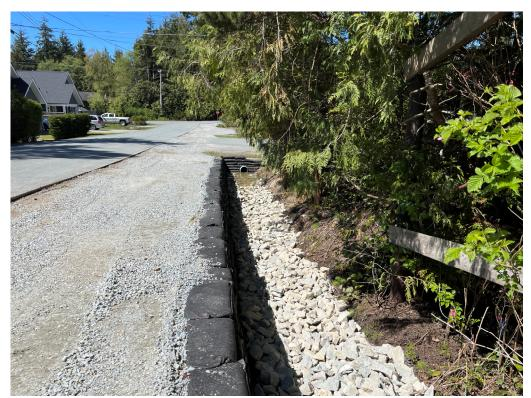
Photo #5 - Rip Rap Ditch Lining Completed
